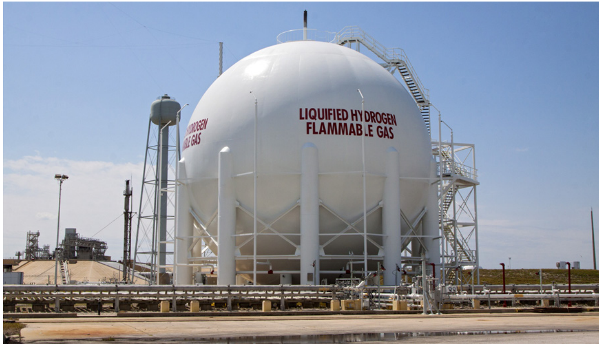
Figure 4-3 – LH 2 storage tank facility at NASA Kennedy Space Centre
