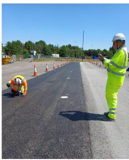
This consisted of two rips each 3.8m wide by 56m long with one gritted at  $0.75 \, \text{kg/m}^2$  and one ungritted. The joint was cut back and sealed prior to laying the second rip and this allowed for extraction of samples to assess the integrity (i.e. voids) at the joint. The material was laid onto an existing surface utilising a Colbond 50 bondcoat applied at  $0.65 \, \text{L/m}^2$ .
