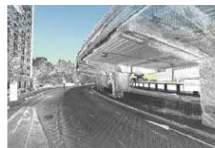
Figure 10. Laser scan image of the M4 Elevated Section
