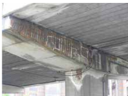
Figure 3. Concrete delamination on crosshead cantilever faces
