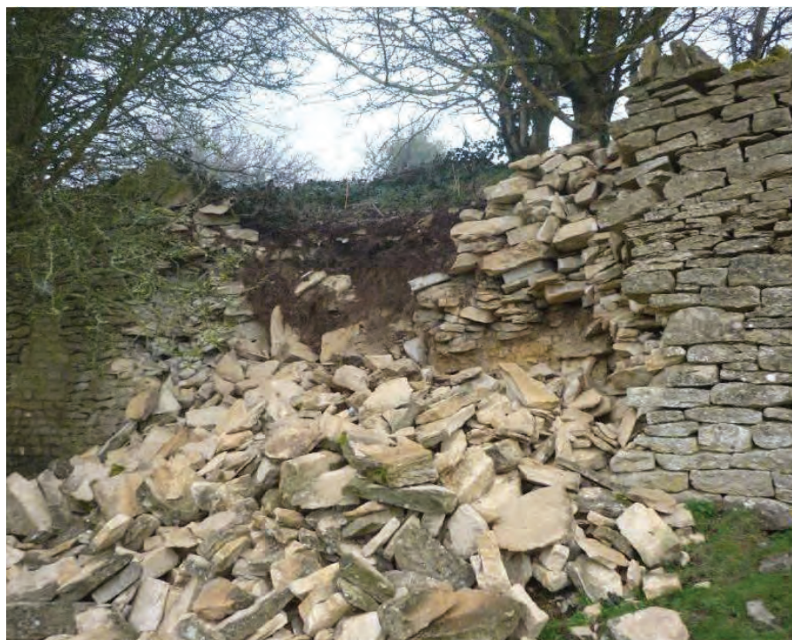
Figure 2. Collapsed Wall at East End, Northleach
