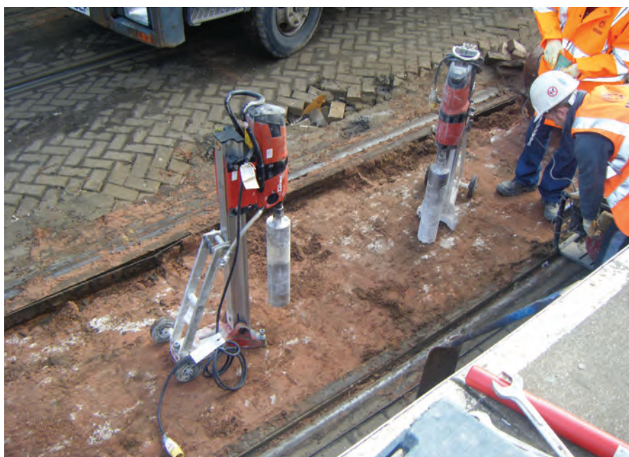
Figure 9. Plate 1-2: Ground investigation set up
