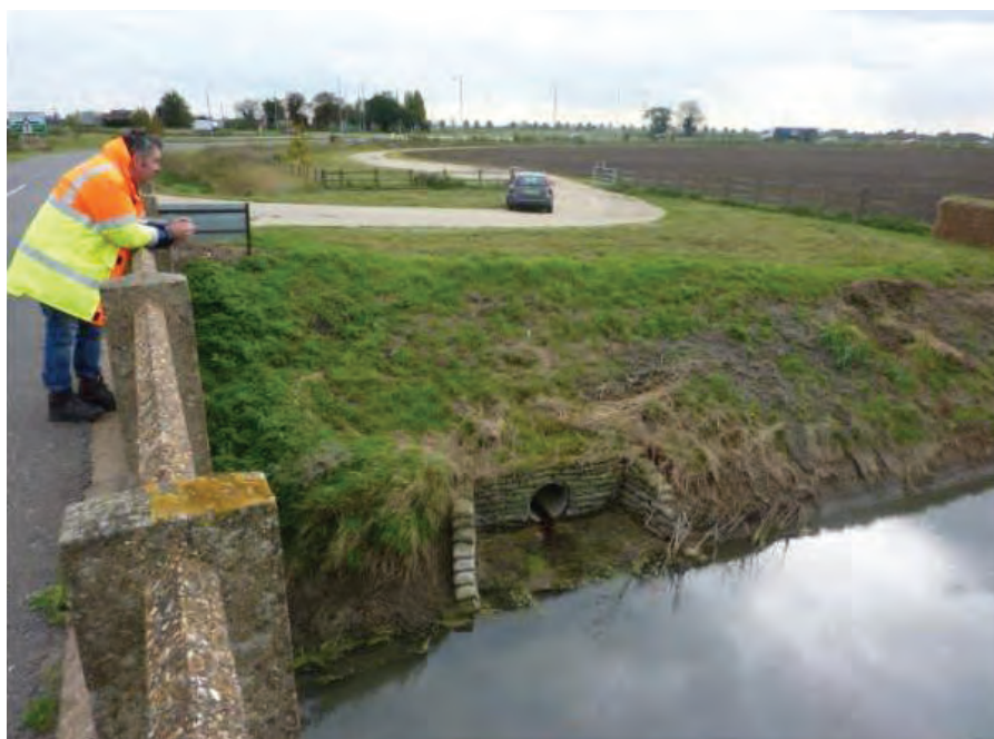
Figure 1. Review of completed road scheme outfall mitigation on Thorney Bypass A47. This would now be required to meet "Good" WFD standards. The reed lined ditch seen in the background (behind access track) is one example of a treatment type not covered in HD 45/09
