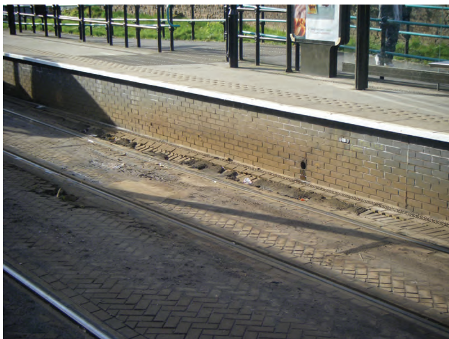
Figure 8. Plate 1-1: Shudehill tramstop in Manchester, showing distressed tracks and surfacing
