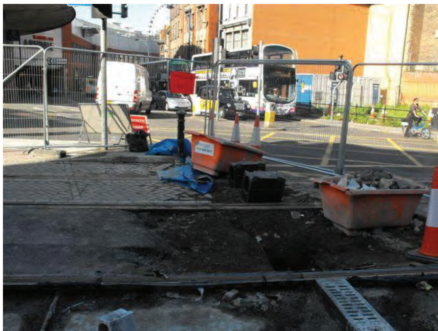
Figure 11. Plate 1-4: Groove drainage upstream of Shudehill ...
