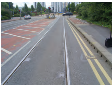
Figure 21. Plate 2-7: Groove drainage upstream of Broadway
