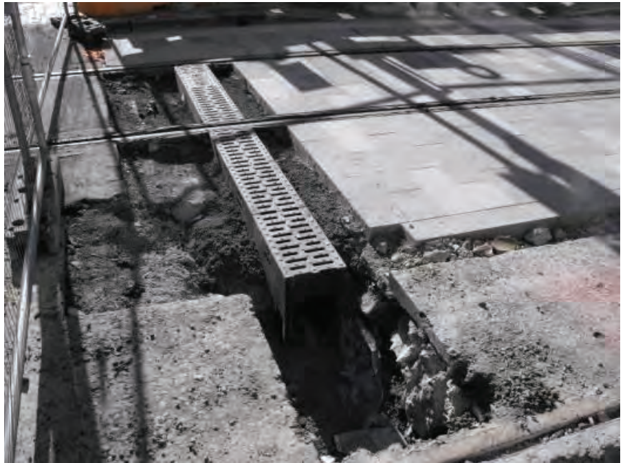
Figure 13. Plate 1-6: Groove drainage at Mosley Street
