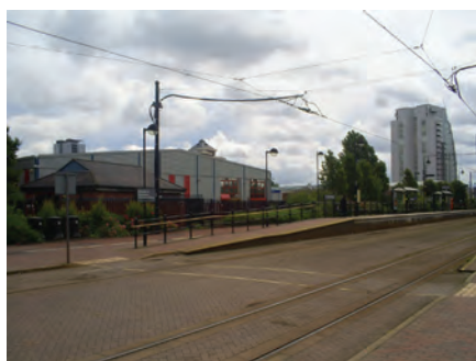
Figure 16. Plate 2-2: Broadway stop, no groove drainage
