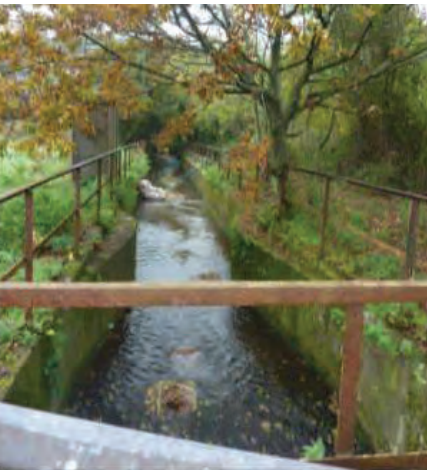
Figure 3. Use of a straw bale (in rear of channel) to filter water quality. No guidance on treatment efficacy exists for similar methods of water quality treatment
