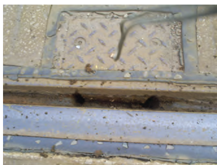
Figure 23. Plate 2-9: Groove drainage upstream of Broadway
