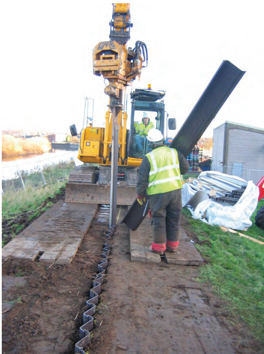
Figure 7. Installing plastic sheet piles to prevent seepage in existing earth flood defence
