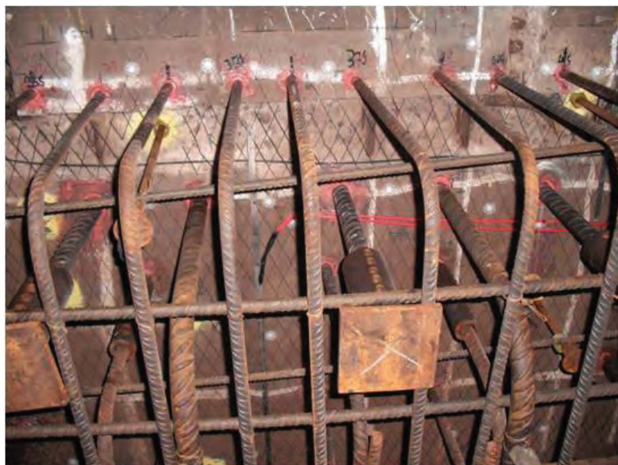
Figure 13. Bars with T-head connection
