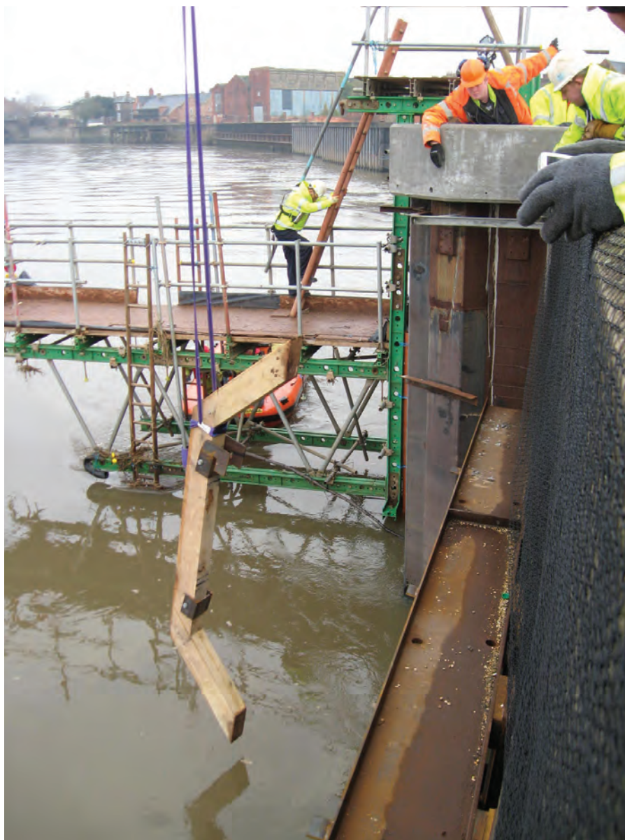
Figure 11. Installing fenders using the quick fixing methods developed by the team
