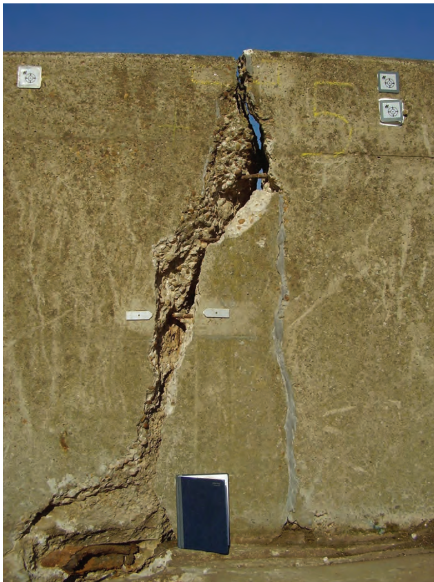
Figure 2. Existing mass gravity flood wall with significant cracking
