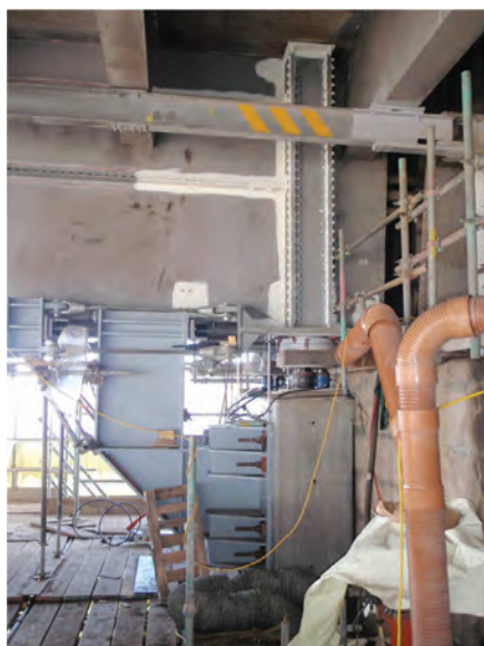
Figure 14. Typical box jacking stiffeners
