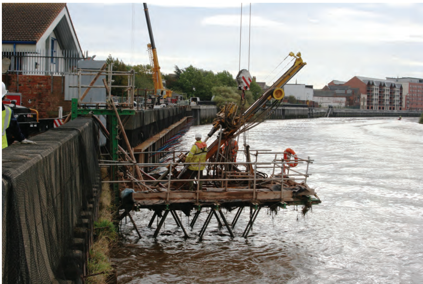
Figure 8. Temporary working platform to allow for installation of ground anchors over the tidal River Trent
