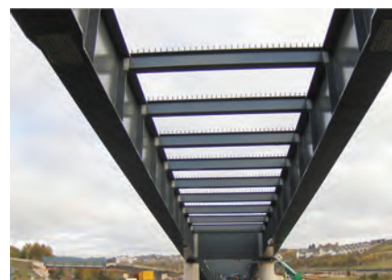
Figure 1. Typical ladder deck geometry (prior to casting deck slab)
