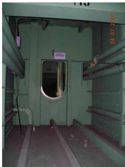
Figure 7. Typical internal view of box girder
