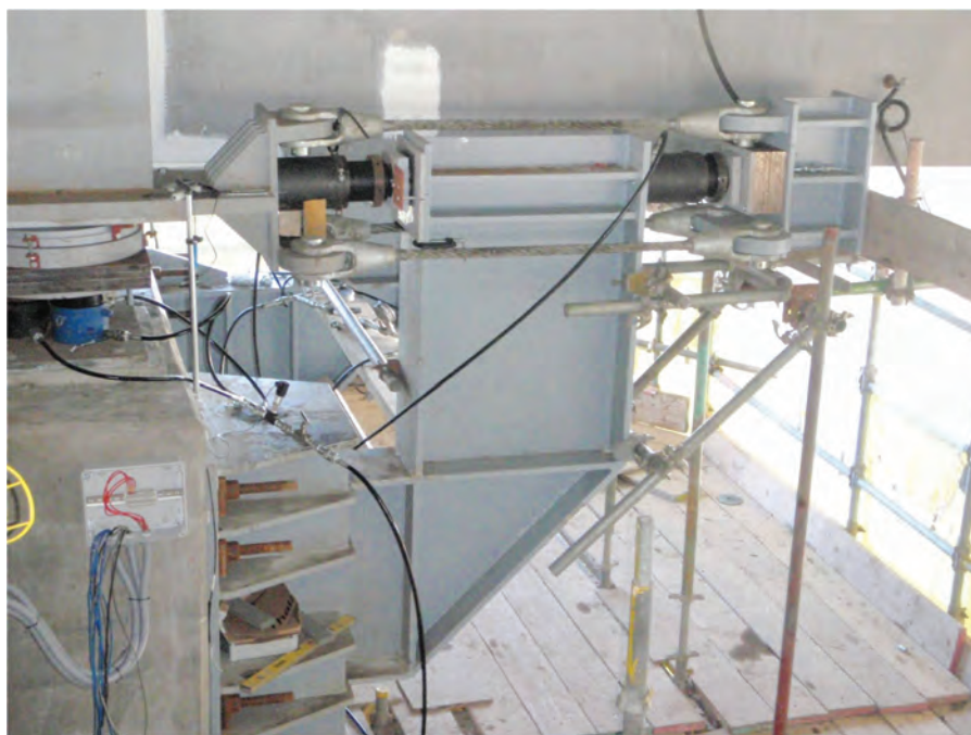
Figure 15. Typical temporary longitudinal restraint
