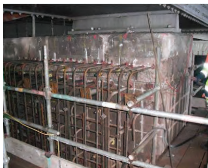
Figure 12. Typical corbel reinforcement and corresponding strut and tie model
