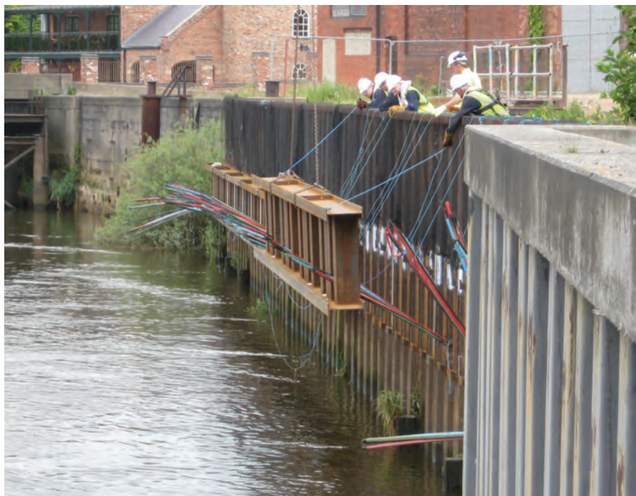
Figure 9. Installing prefabricated waling beam sections – packers are required between the beams and the existing piles to ensure an even transfer of loads
