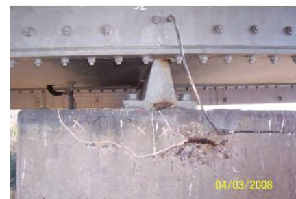
Figure 5. Typical rocker bearing
