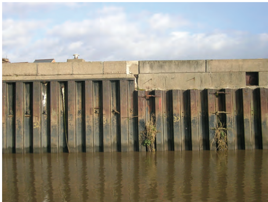
Figure 5. Existing anchored sheet pile walls in visually poor condition
