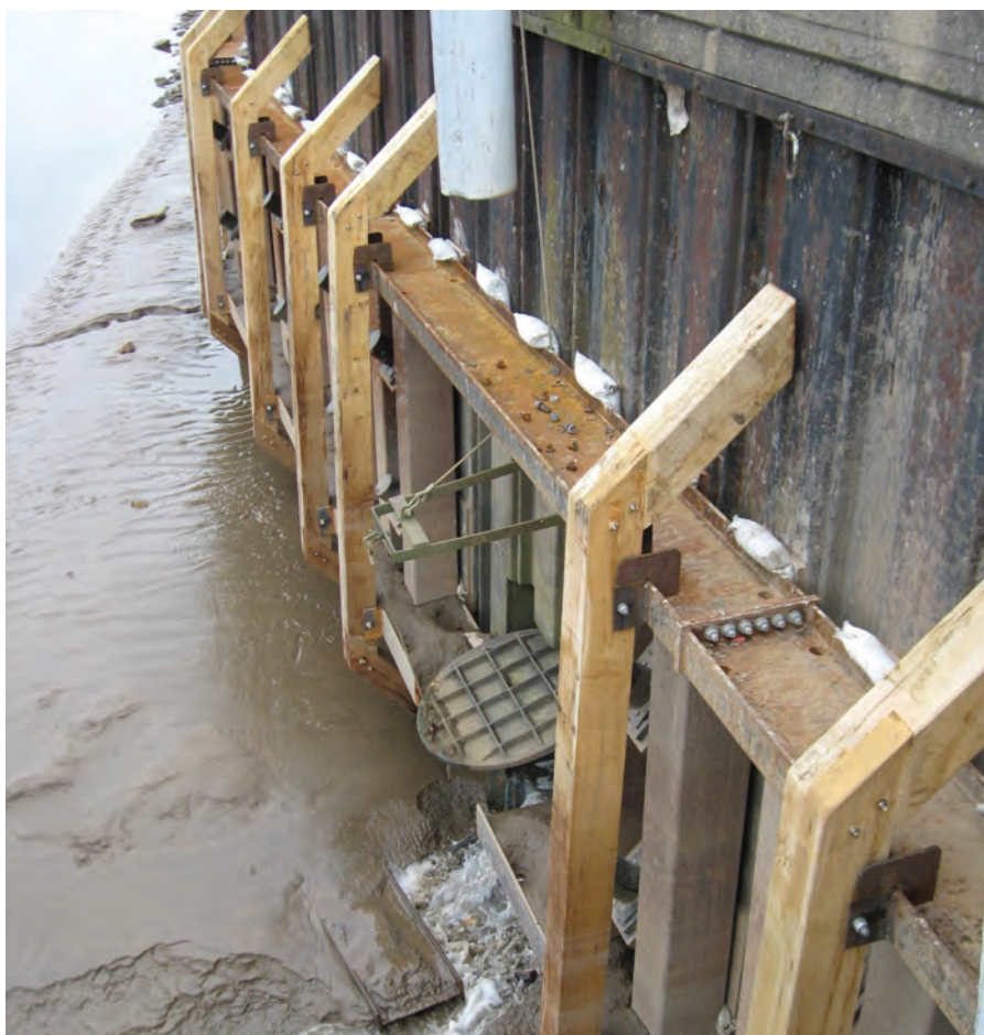
Figure 10. Completed section showing waling beam, grout packers and fenders
