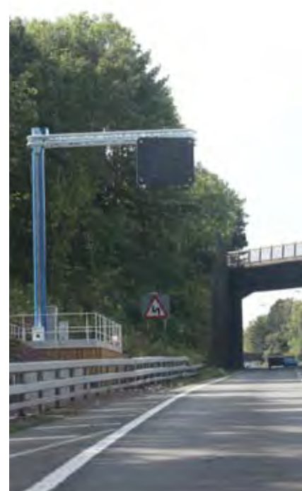
Figure 3. Verge signal rotated to operational position (M4 Newport)
