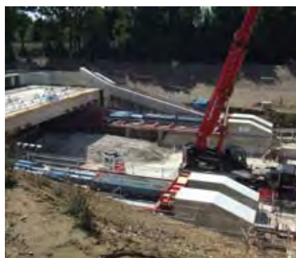
Figure 11. Rear jacking station during installation of the first deck unit operations
