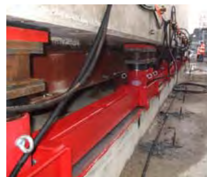
Figure 9. 3,200t sliding system on prefab yard
