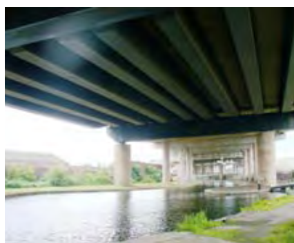
Figure 1. Typical steel-concrete composite box girder spans
