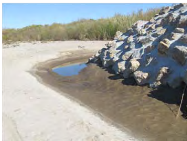
Figure 10. Upstream progression of scour
