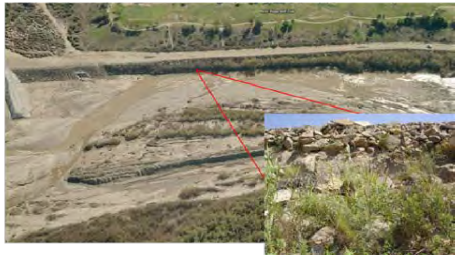
Figure 1. Typical toe scour along bank
