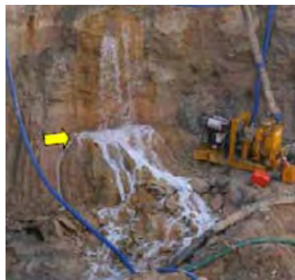
Figure 3. Example of piping failure
