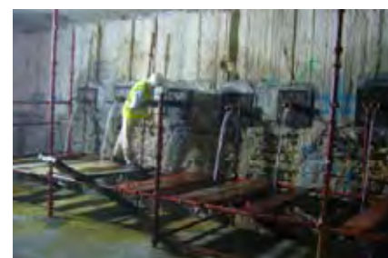
Figure 11. Installation of drain pipes installed below the adit invert of annex 3
