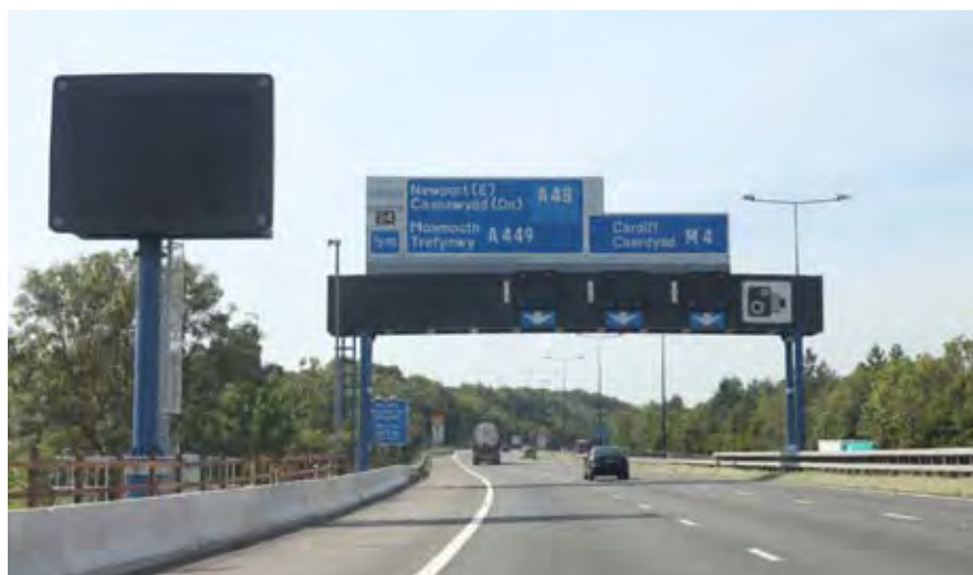
Figure 5. Combination of existing variable message signs in verge and on gantries (M4 Newport)
