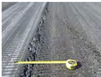
Figure 2. Cracking/tearing of wearing course on Runway 9/27
