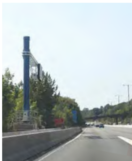
Figure 4. Verge signal rotated away from carriageway to facilitate maintenance (M4 Newport)
