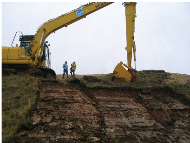
Figure 6 - Removing turves from the Boston Spa site with a modified bale-cutting bucket in spring 2006
