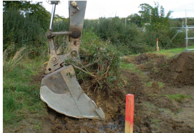
Figure 3 - Placing a hedge section in the receptor trench, which had a slow-release fertiliser and water-retaining gel
