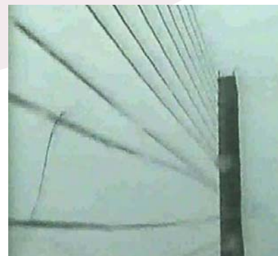
Figure 1- Large amplitude stay cable vibrations
