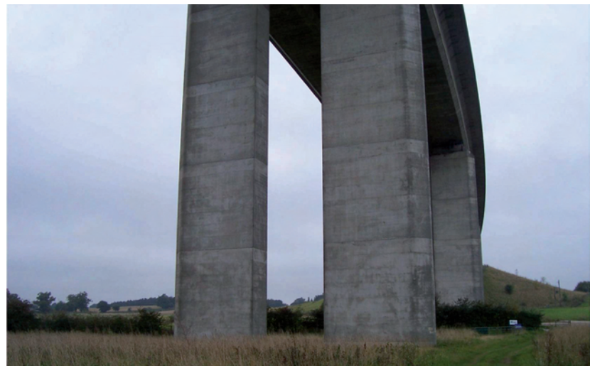
Figure 1 - (ii) Photo taken at Pier 5, where the height of the pier from the top of pile cap is 34.5m
