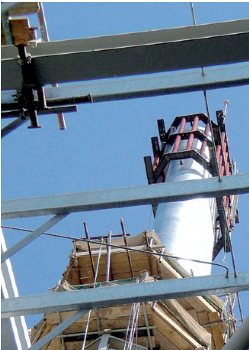
Figure 11 - Temporary device to suppress vortex shedding on the spire during construction of the spire and installation of its tuned mass dampers
