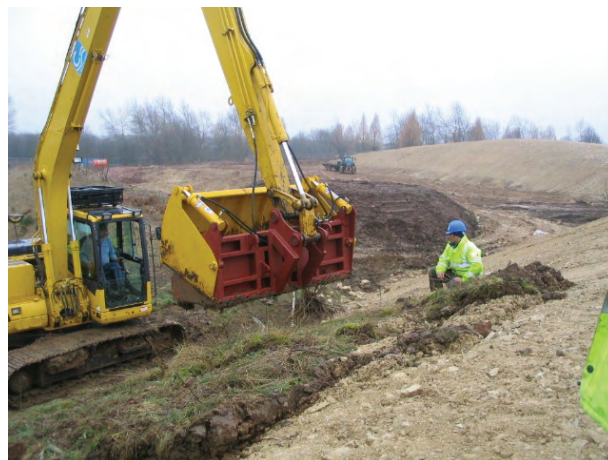
Figure 7 - Placing turves on the new landscape bund at Boston Spa
