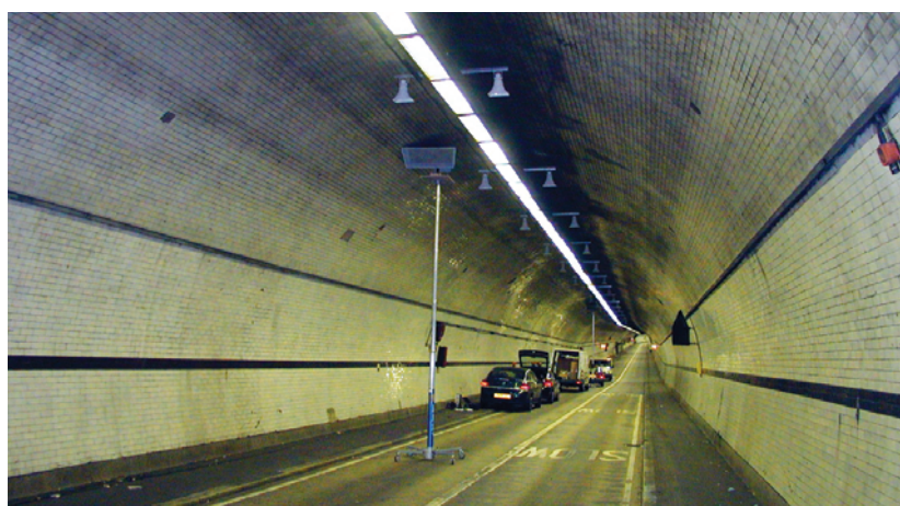
Figure 4 - A trial section of speakers in the Rotherhithe Tunnel.
