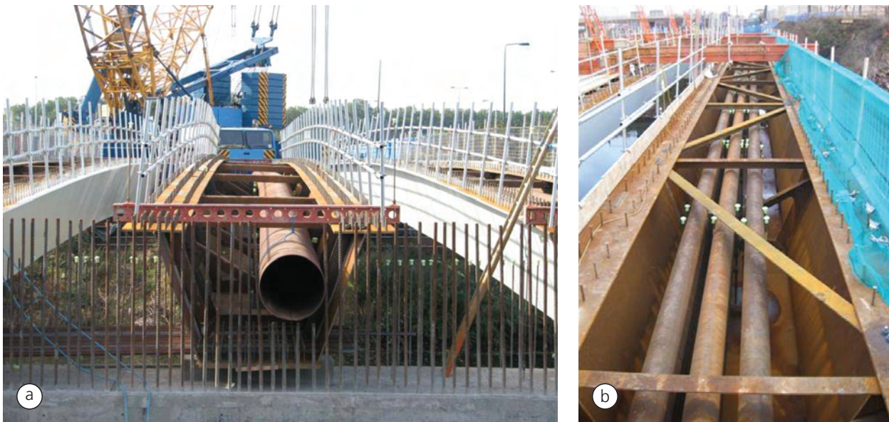
Figure 5 - (a) Twisted box under eccentric load; (b) Addition of plan bracing
