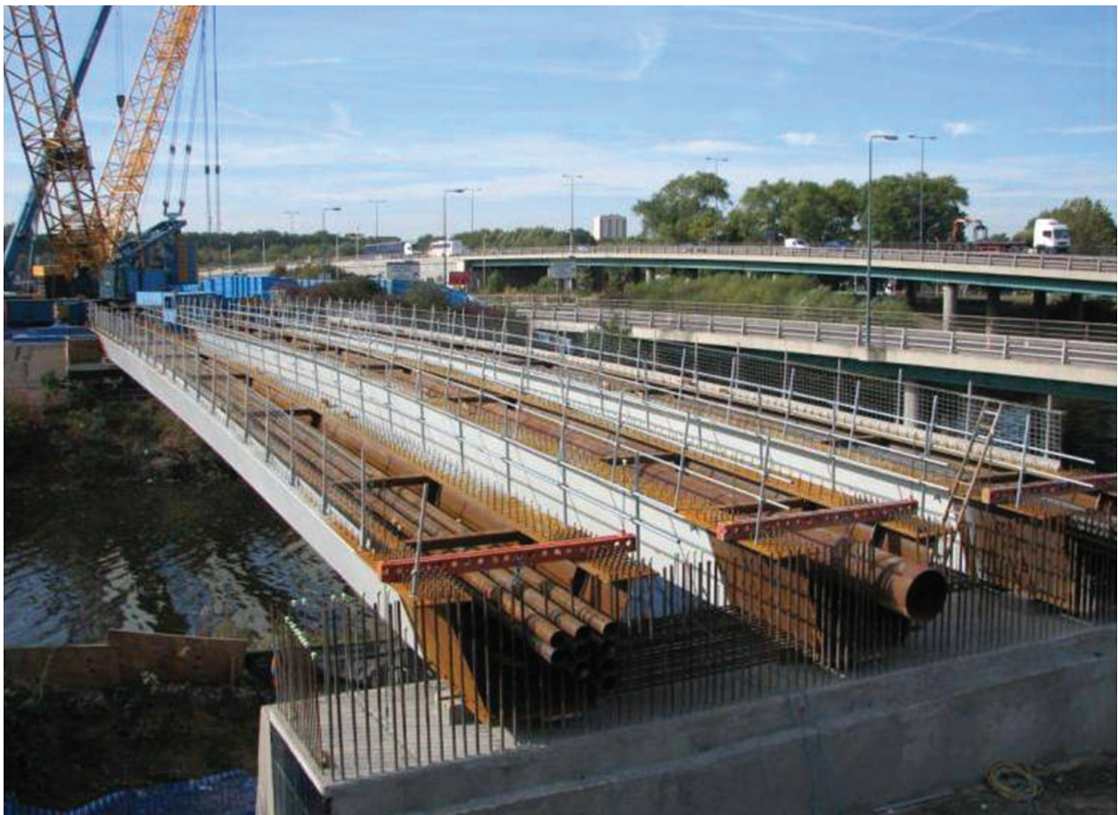
Figure 2 - Bridge H01 prior to deck slab construction
