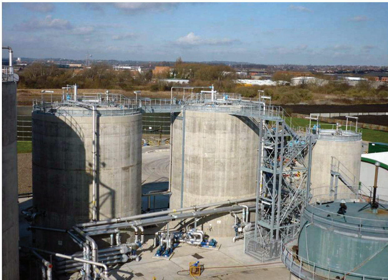
Figure 3 - APD at Derby STW. The two tanks in the middle are APD 1 and APD 2, with their heat exchangers and recirculation pumps just in front. The smaller tank to the right is the APD BT. You can just see the edge of one of the larger MADs on the left of the frame. The green tank in the foreground to the right is the gas holder.
