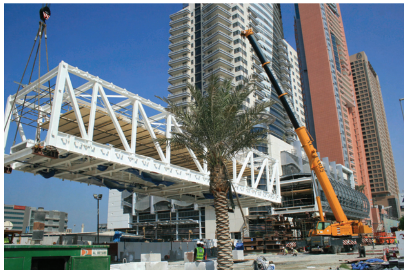
Figure 15 - Footbridge erection using mobile crane
