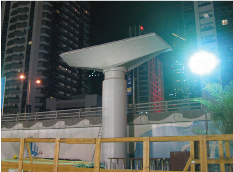
Figure 5 - Typical standard pier arrangement during construction
