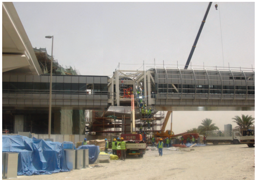
Figure 17 - Steel extensions above pier heads at footbridge junctions during construction
