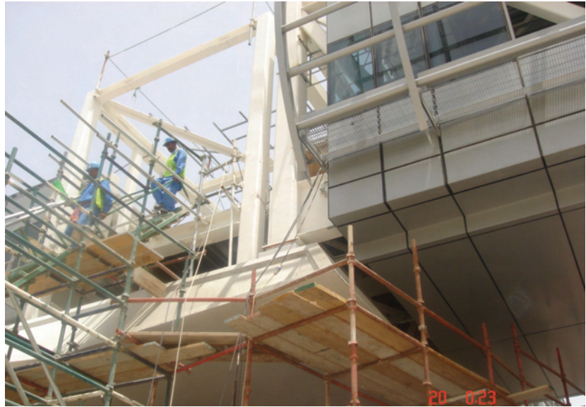
Figure 16 - Steel extensions above pier heads at footbridge junctions during construction
