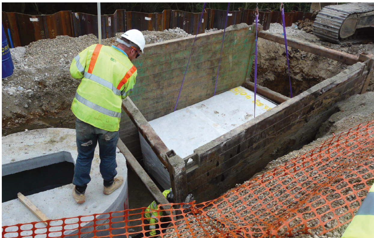
Figure 3 - Installation of geo-cellular tank
