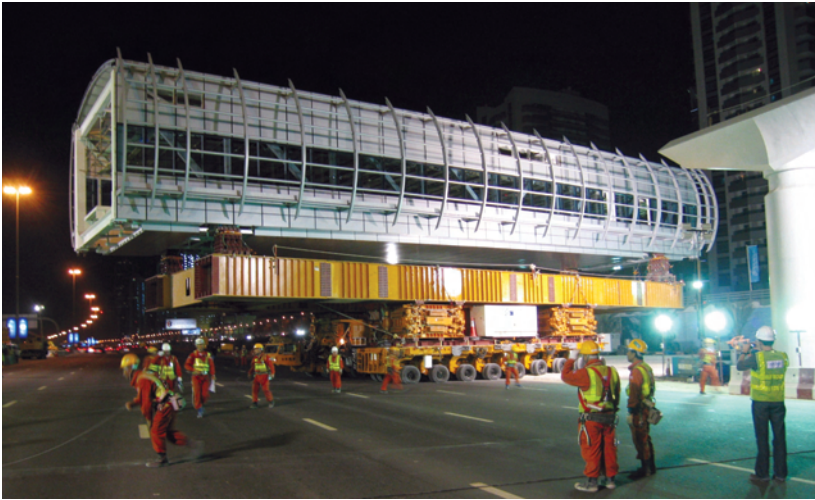
Figure 14 - Footbridge supported on SPMT
