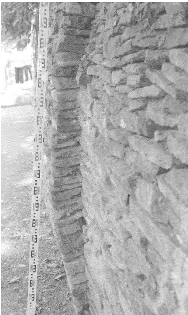
Figure 5 - Deformed wall
