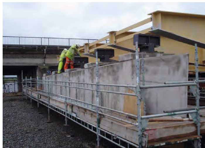
Figure 15 - Nose approaching launch bearings at a pier prior to touch-down
