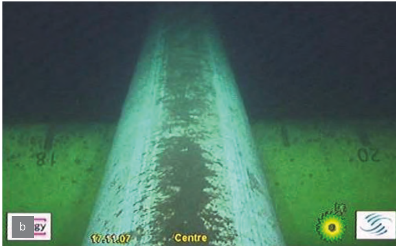
Figure 38 - OOS surveys – (a) Survey Data comparison, (b) Pipe movement on initiator
