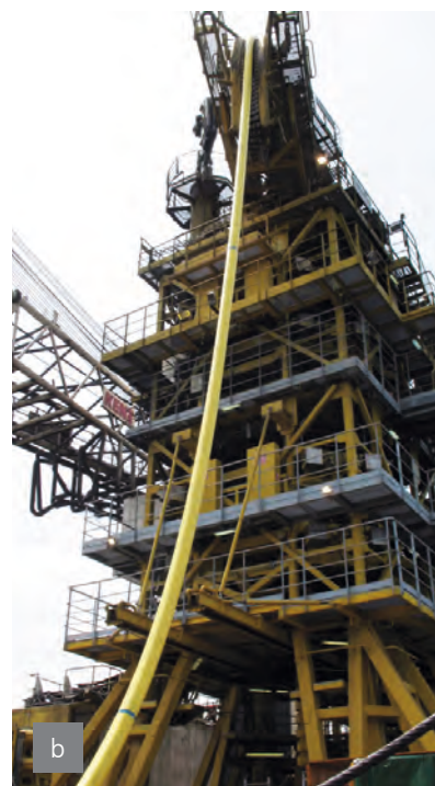
Figure 23 - Installation of subsea structures (a) and flexible spurs (b)
