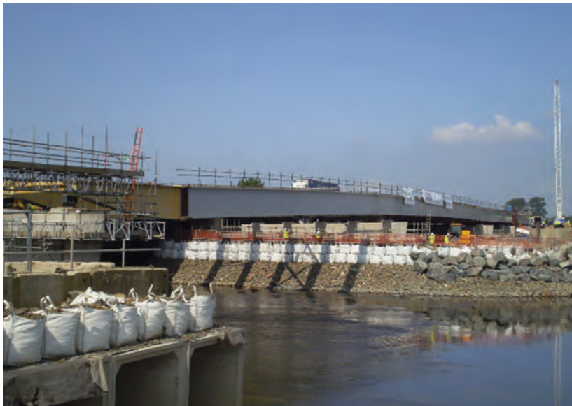
Figure 6 - View of the launch showing significant leading span cantilever deflection and temporary cofferdam/island around an intermediate pier
