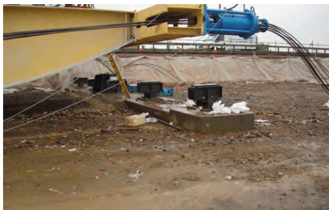
Figure 13 - View of tail, temporary land base, launch bearings and strandjack launch system
