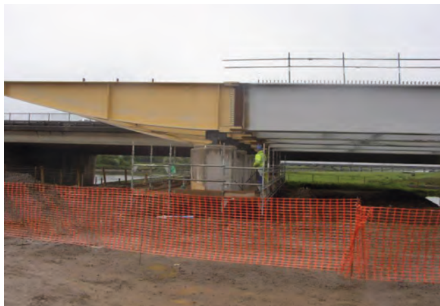
Figure 12 - Touch down at an intermediate pier position
