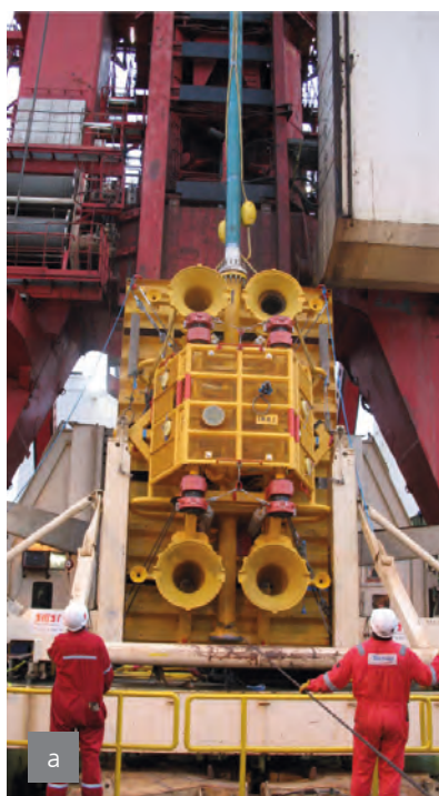
Figure 23 - Installation of subsea structures (a) and flexible spurs (b)
