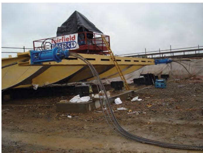
Figure 20 - Strand-jack launching system with stiff cross beam transferring loads to tail beam ends - monitoring station under cover in background
