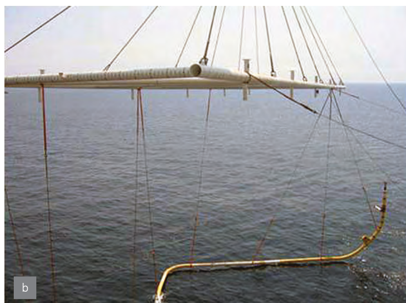
Figure 31 - Rigid spool installation
