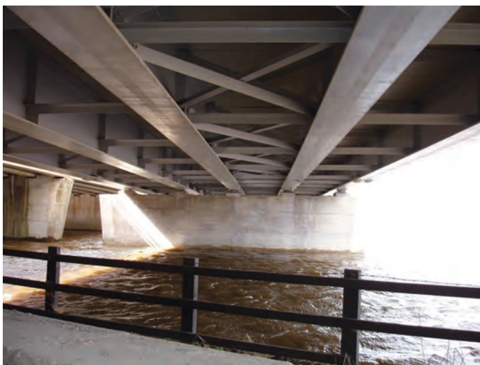
Figure 17 - View showing launch track marks on bottom flanges and plan bracing left in place
