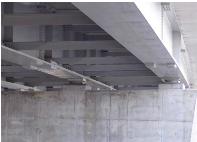
Figure 22 - Split bottom flange splice plates
