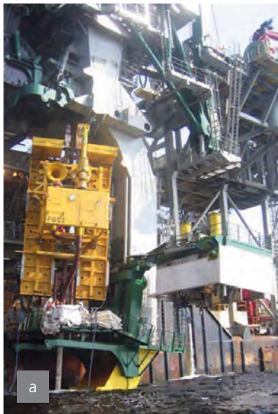
Figure 28 - Installation of FTA and ILT structures
