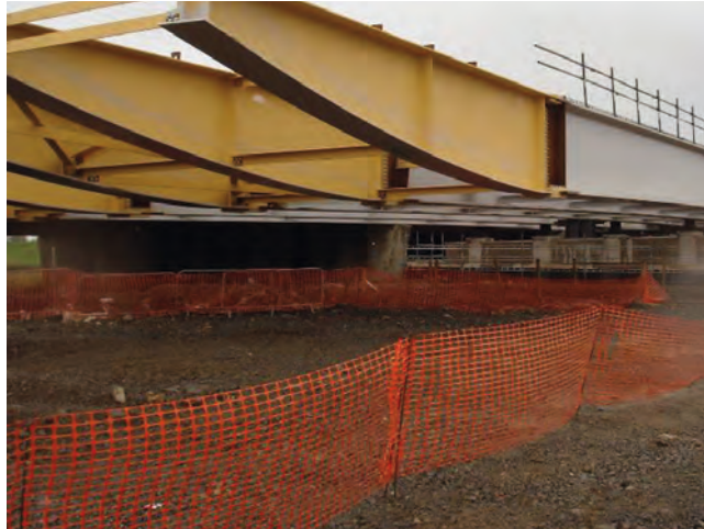
Figure 11 - View of leading span and nose during the launch
