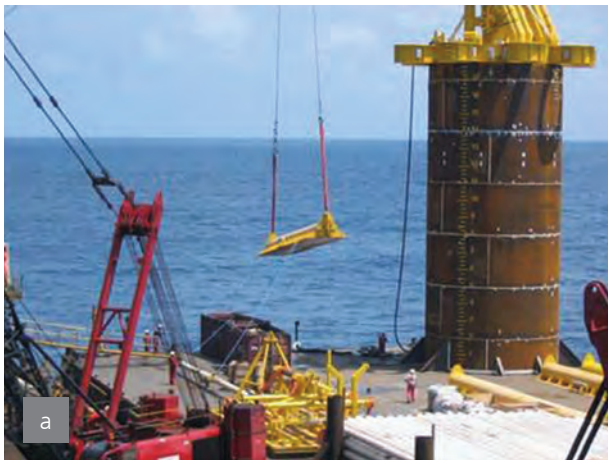
Figure 30 - Sleeper deployment and pipelay over a sleeper
