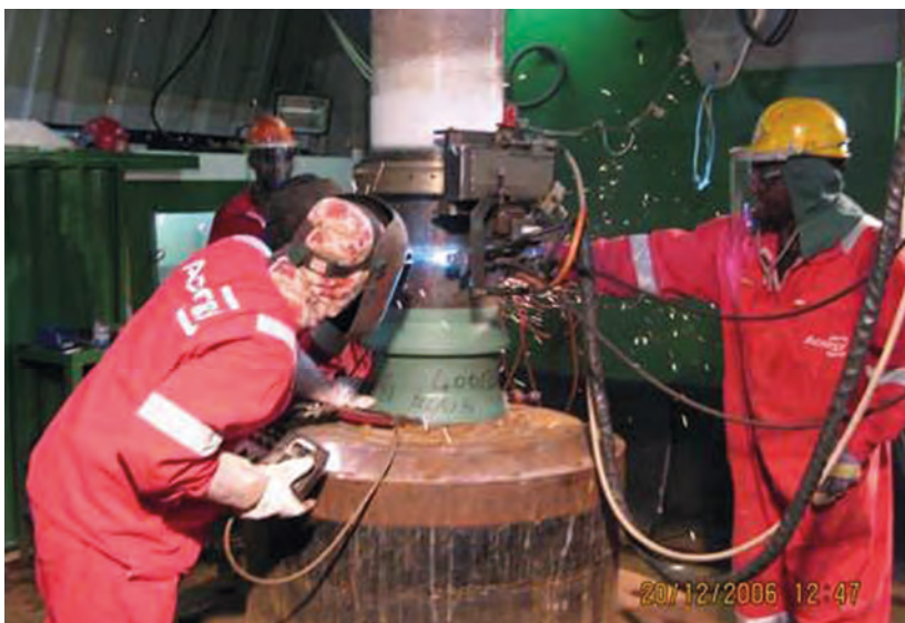
Figure 27 - First weld performed on flowline
