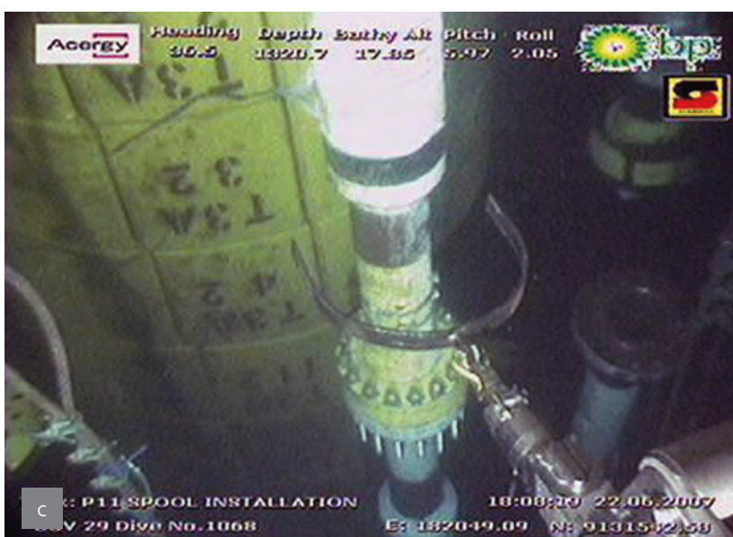
Figure 32 - Matis flanged spool connection
