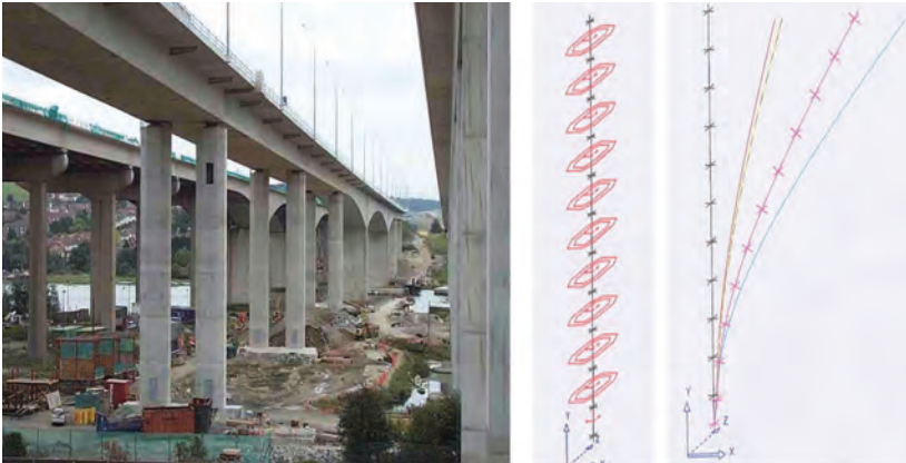
Figure 9 - Non-linear analysis of slender piers (deflected shapes shown for various load cases)
