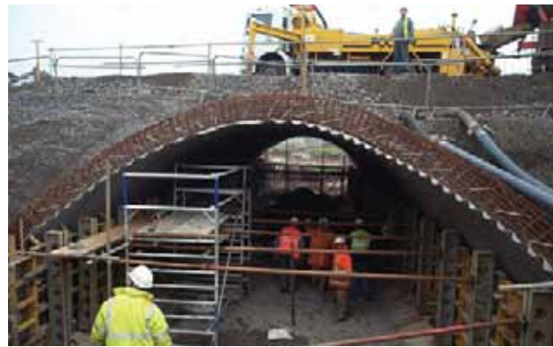
Figure 10 - Fixing of reinforcement to top half of collar beam
