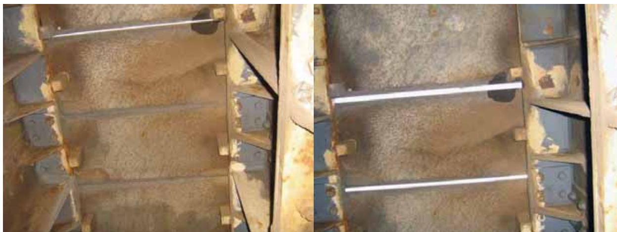
Figure 11 - Opening and closing of gaps in the plate train (viewed from below)
