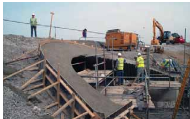
Figure 12 - Collar beam concrete in place
