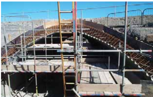
Figure 11 - Scaffold arrangement for access and for propping of corrugated steel during concrete pour
