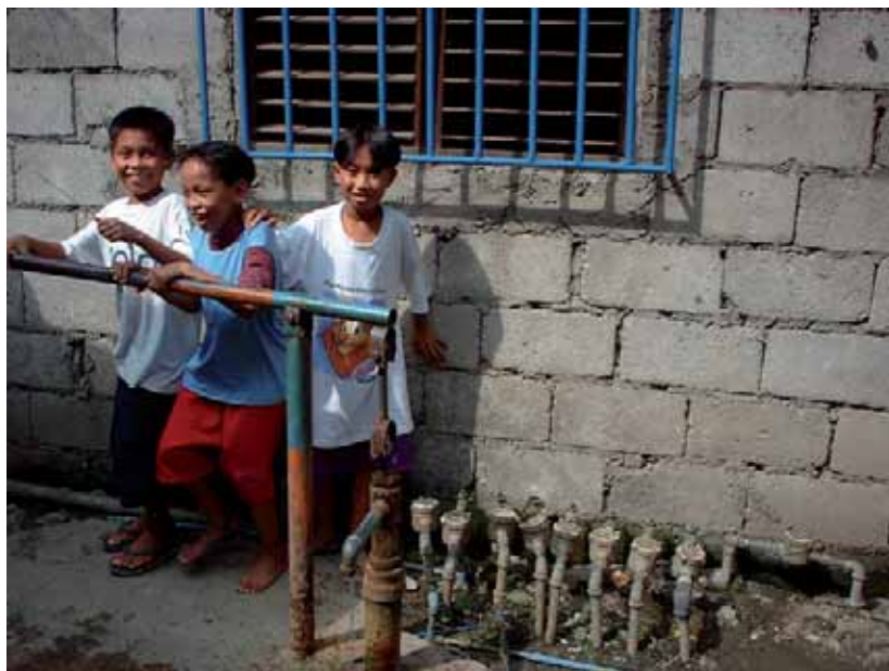
Figure 2 - Piped water through remote meters replacing potentially contaminated groundwater in a slum in Manila, the Philippines (Photo: Franceys)
