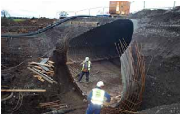
Figure 9 - Fixing of reinforcement to bottom half of collar beam
