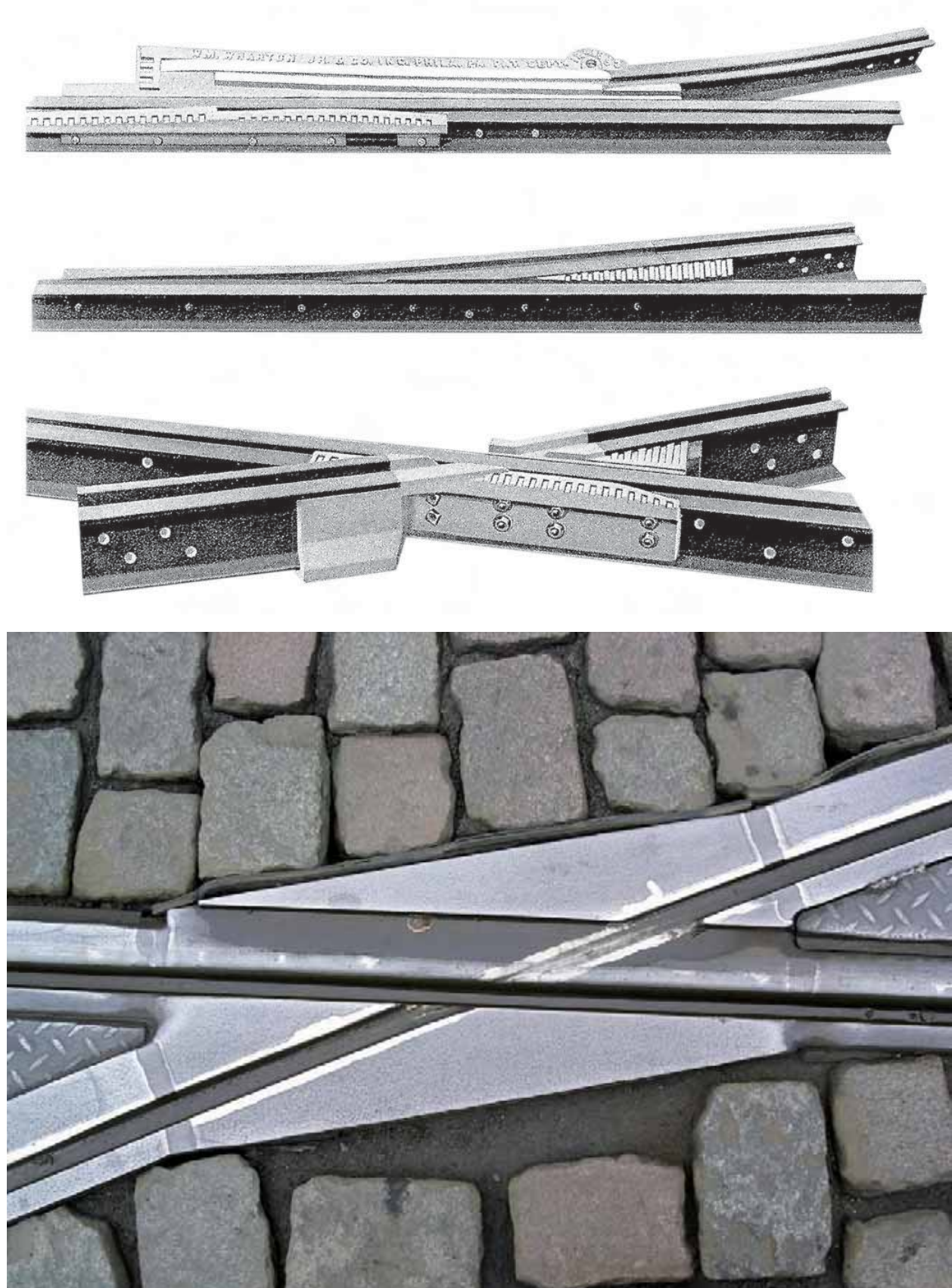
Figure 4 - The Wharton Unbroken Main Line Construction, one of the earliest lift-over crossings, together with its modern equivalent. The latter indicates some wear of the main rail head
