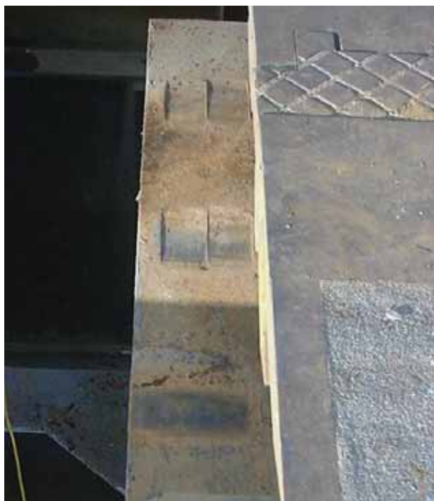
Figure 7 - Wear in top flange of track beams
