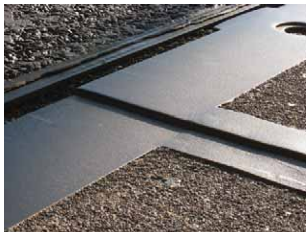
Figure 9 - Misalignment between adjacent shuttle plates
