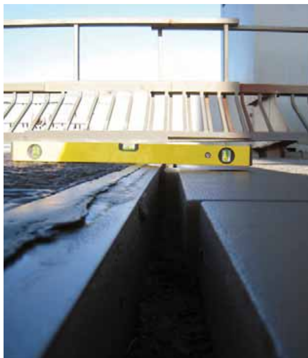
Figure 10 - Misalignment of tongue plates
