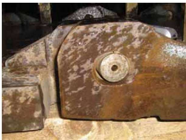
Figure 8 - Wear in hinge pin hole and misalignment of the pin
