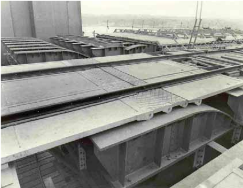
Figure 4 - Roller shutter joint installation (early 1960s)
