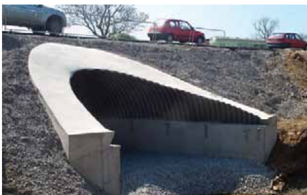
Figure 13 - Finished collar beam
