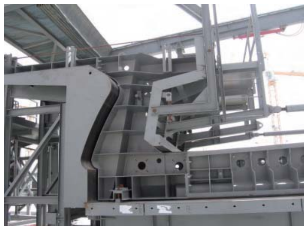
FIGURE 13. THE STEEL FORMWORK USED FOR SEGMENTS CASTING, SHOWING THE TENDONS' FIXED POINTS
