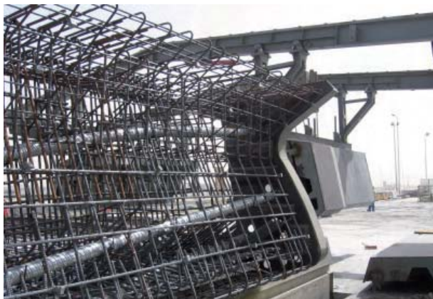
FIGURE 15. STEEL CAGE OF ONE SEGMENT AND THE DUCTS IN POSITION, BULK-HEADS IN POSITION, WHILE INNER SHUTTER BEING SLIDE INTO THE DECK
