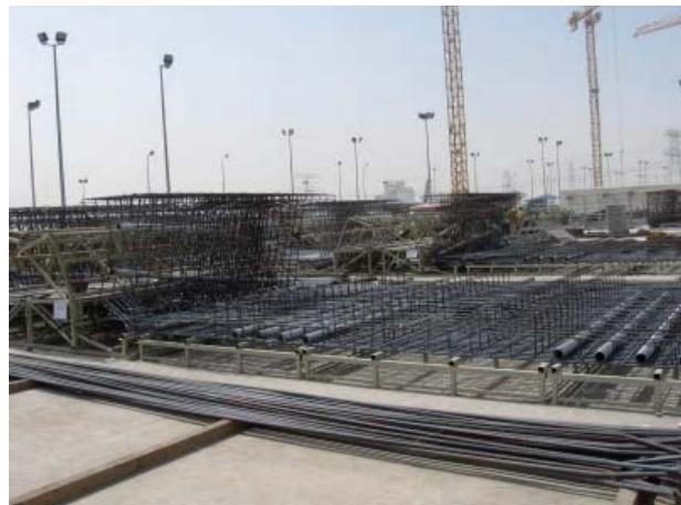
FIGURE 12. ASSEMBLY AREA FOR SEGMENTS' REINFORCEMENT, REINFORCEMENT CAGE IS READY TO BE MOVED TO CASTING MOULD
