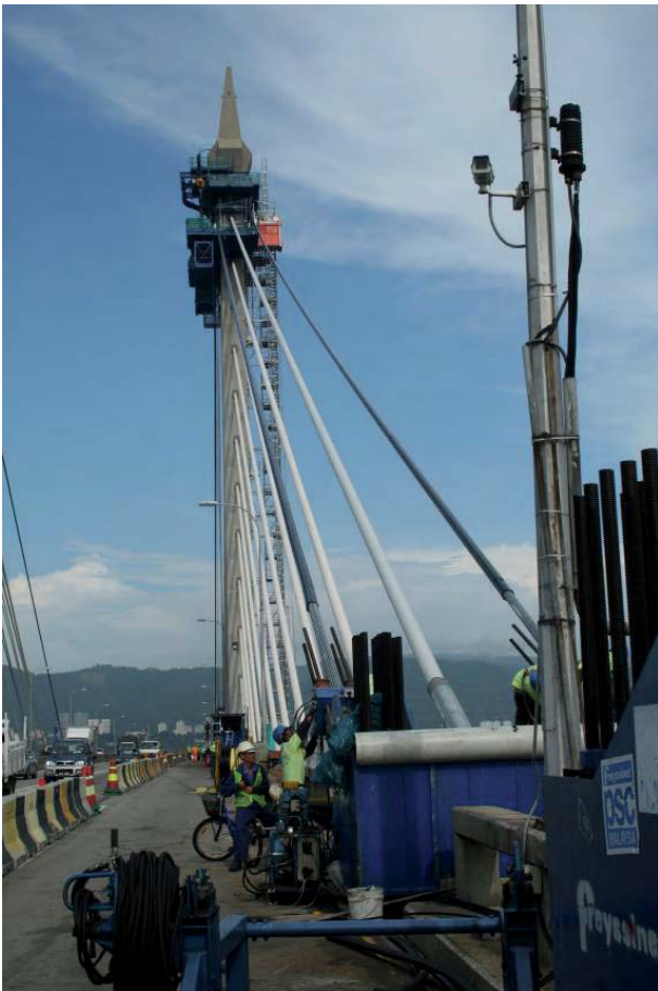
FIGURE 18. TYPICAL TEMPORARY WORKS REQUIRED TO REPLACE A SET OF SIMILAR CABLES
