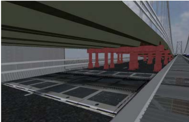
FIGURE 15. FORTH EXPANSION JOINTS WITH TEMPORARY FLYOVER
