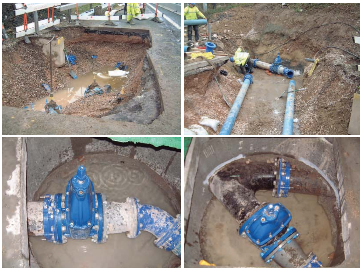
FIGURE 3. SUSPECTED LOCATION OF LEAK - WORKS CARRIED OUT IN FEBRUARY 2007 SHOWING PIPING AND VALVE LAYOUTS AT THE EAST PORTAL
