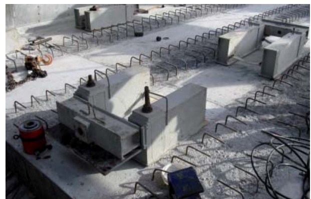
FIGURE 18. STEEL BRACKETS FOR APPLYING TEMPORARY PRESTRESS
