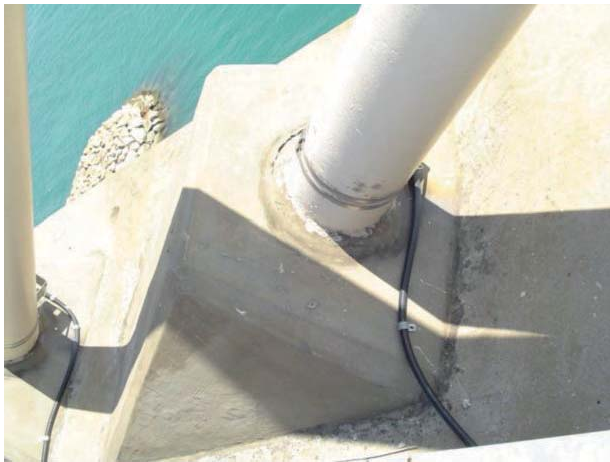
FIGURE 5. EXISTING CABLE ANCHORAGE: (II) DETERIORATION OF RUBBER GASKET
