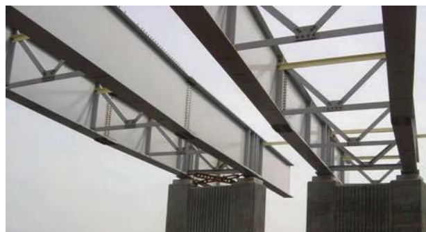
FIGURE 1. BRACED BEAMS IN PAIRS PRIOR TO CONCRETING
