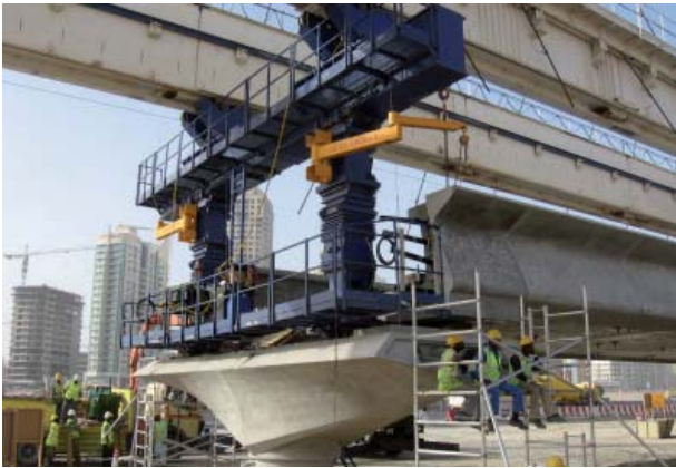
FIGURE 8. GANTRY'S FRONT SUPPORT RESTING ON A PIER, ERECTED DECK IN POSITION AFTER ITS PRESTRESSING IS COMPLETED
