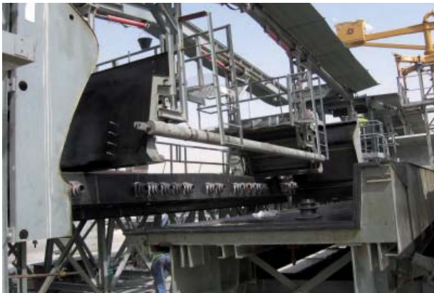
FIGURE 14. INNER SHUTTER AND BULK-HEAD FOR A MID-SPAN SEGMENT
