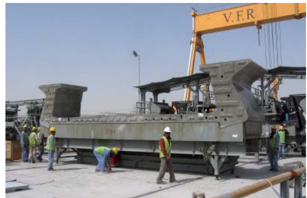
FIGURE 16. ONE SEGMENT AFTER CONCRETE HARDENING WHILE STILL ON THE SOFFIT SHUTTER, READY TO BE MOVED TO STORAGE YARD
