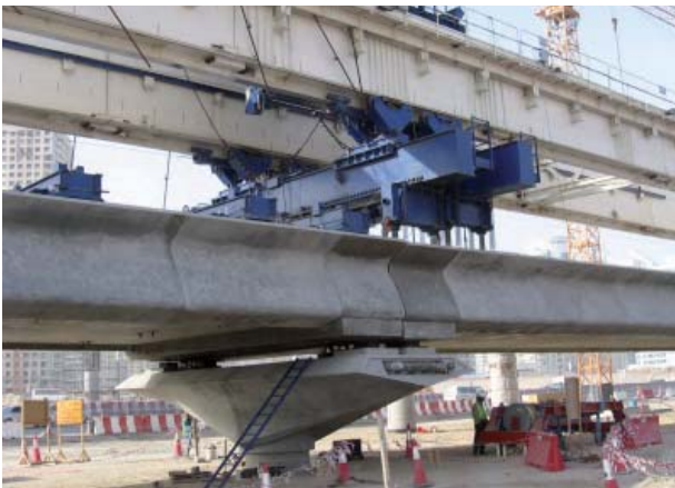
FIGURE 9. GANTRY'S REAR AND AUXILIARY SUPPORTS RESTING ON DECK'S GIRDERS
