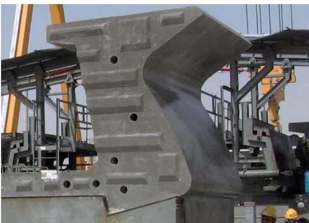
FIGURE 11. SHEAR KEYS
