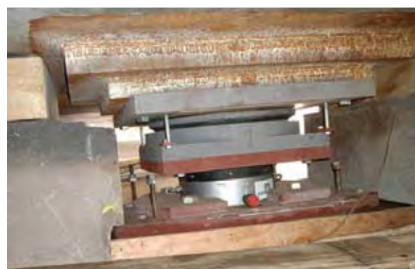
FIGURE 14 "KEEP" PLATES TO HOLD JACK IN POSITION AND FIX BEARING TO JACK
