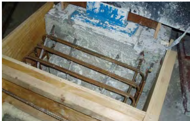
FIGURE 15 EXTENSION OF BEARING PLINTHS
