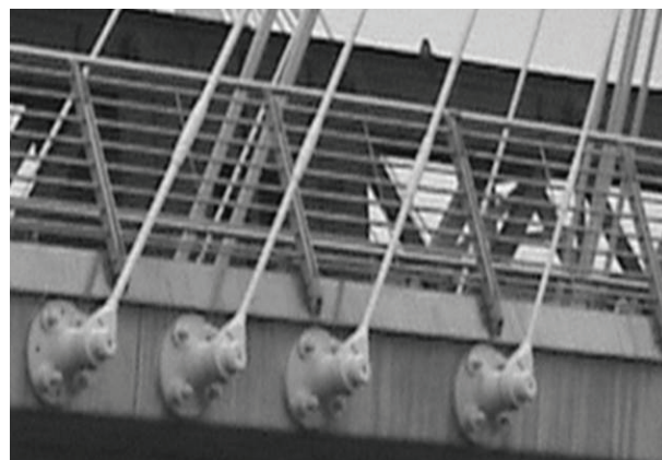
FIGURE 6 CABLE STAY ANCHORAGE
