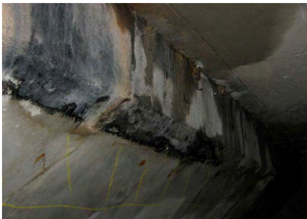
FIGURE 2 RESULT OF LEAKING DECK JOINT.
