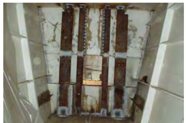
FIGURE 19 FINAL STRENGTHENING ARRANGEMENT
