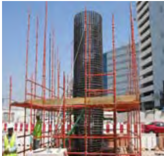
FIGURE 8 CONSTRUCTION OF TYPICAL PIER ON A MONOPILE FOUNDATION
