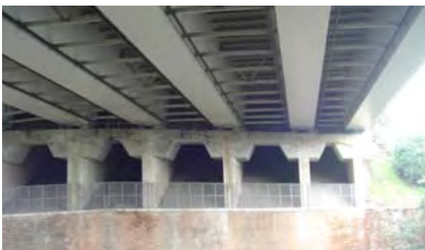
FIGURE 16 STRENGTHENING TO SUBSTRUCTURE
