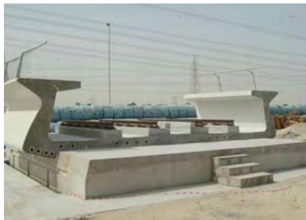
FIGURE 6 PROTOTYPE DECK SEGMENT ILLUSTRATING TYPICAL SECTION AND FINISH
