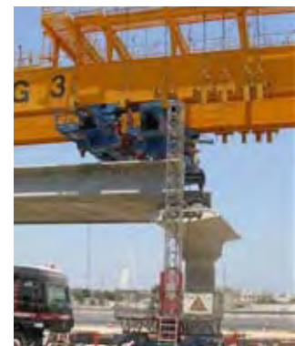
FIGURE 14 HIGH ECCENTRICITY OF TEMPORARY LOADING FROM OVERHEAD GANTRIES
