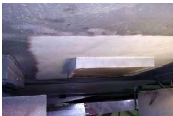
FIGURE 11 EXISTING BEARING PLATE BENEATH BOTTOM FLANGE
