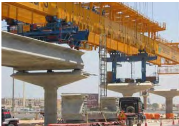
FIGURE 10 USE OF OVERHEAD GANTRIES TO CONSTRUCT TYPICAL VIADUCT SECTIONS
