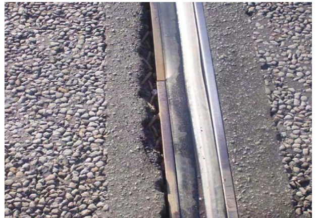
FIGURE 3 FAILURE OF METAL RUNNER FIXING IN NOSING.
