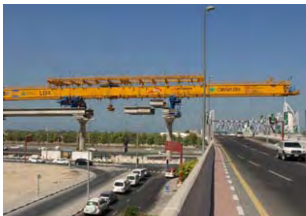
FIGURE 11 USE OF OVERHEAD GANTRIES TO CONSTRUCT TYPICAL VIADUCT SECTIONS
