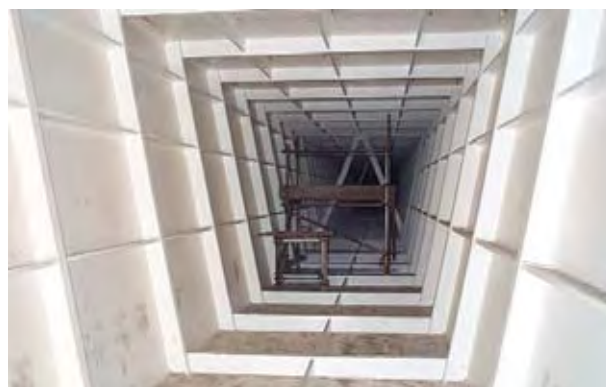
FIGURE 2 INTERNAL STIFFENING TO BOX
