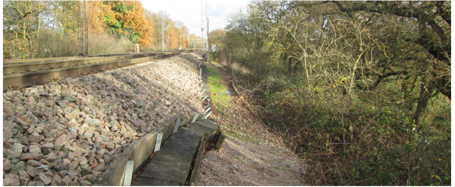
B) 49m 78ch Up Large dip in cess walkway and associated track dip
