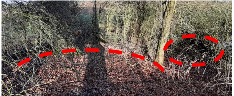
E) 49m 76ch Down Historic toe bulge blocking toe ditch causing ponding at slope toe
