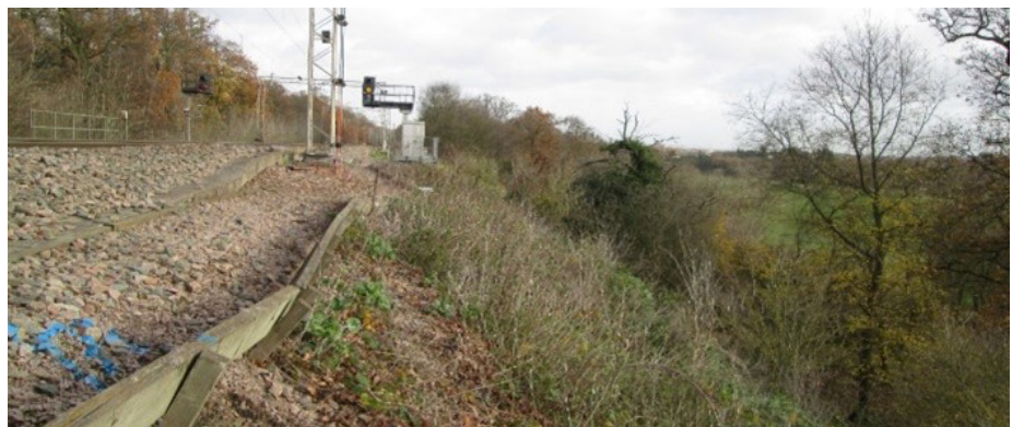
A) 49m 71ch Up Exposed sleeper ends, ballast spalling down slope and failing cess
