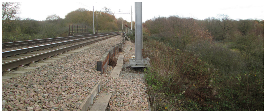
D) 50m 15ch Up Sleeper ends exposed, poor cess condition. A small king post retaining wall has been constructed to retain ballast at this location.
