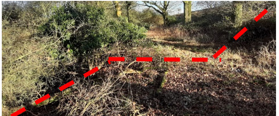
F) 50m 05 to 12ch Down Toe berm on slope – possible historic stabilisation?
