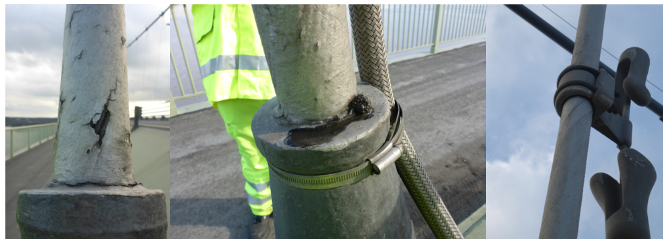
Figure 6: Typical hanger defects
