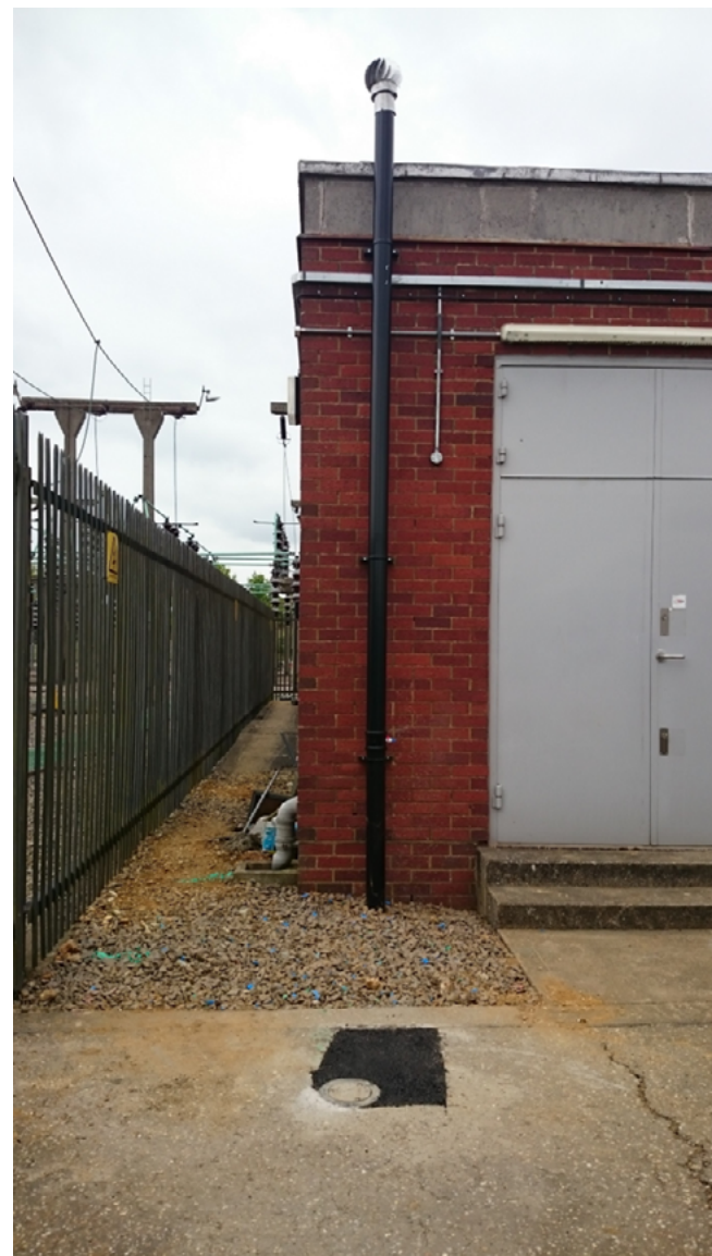
Figure 4: Venting cowls installed around the perimeter of the relay room building
