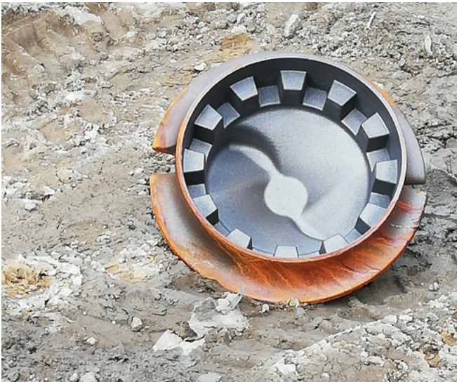
Figure 3: The tip of the Fundex pile.
