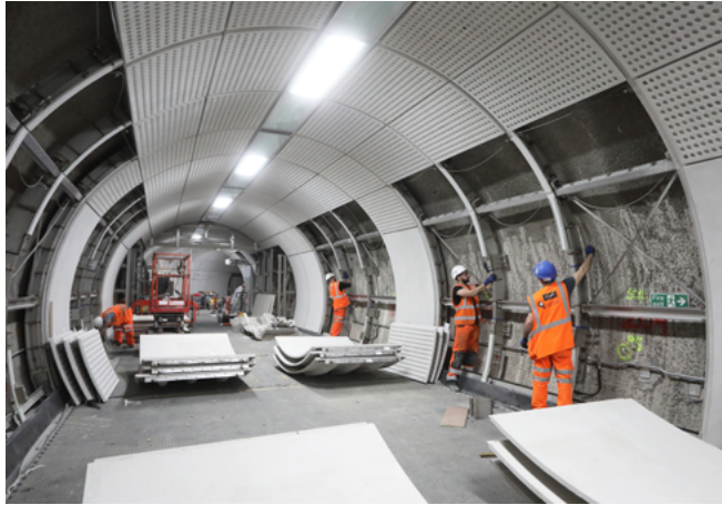
Figure 9: Installation of GFRC cladding in a station tunnel © Crossrail.
