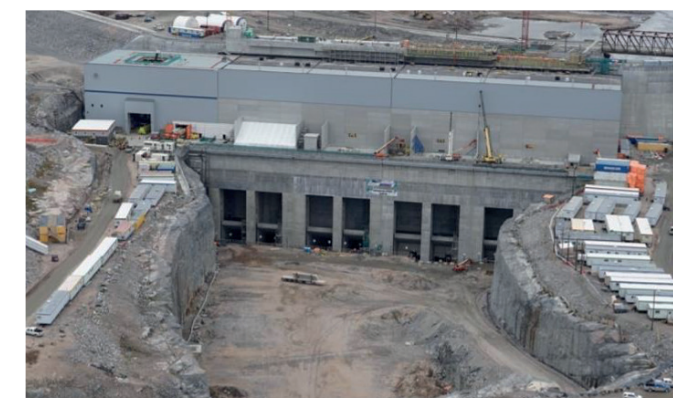
Figure 8: Tailrace prior to watering up (September 2018).
