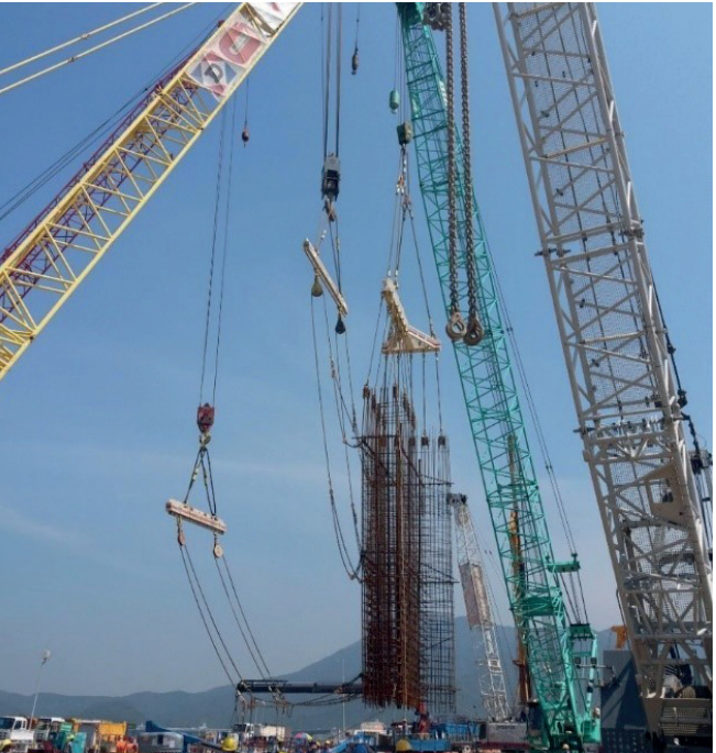
Figure 5-7: Y-panel rebar cage lifting operation
