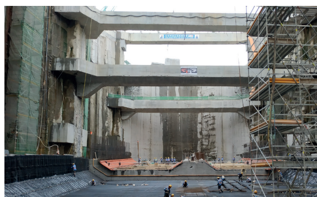
Figure 4-4: Typical ELS cross section showing lateral support
