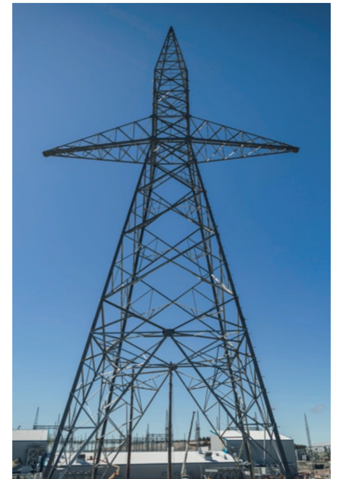
Figure 16: HVDC transmission tower
