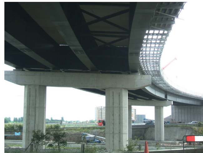
Figure 1: Typical curved in plan multi-girder bridge
