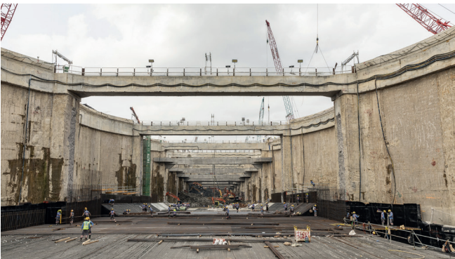
Figure 3-4: Clear space below the lowest strut for tunnel box construction
