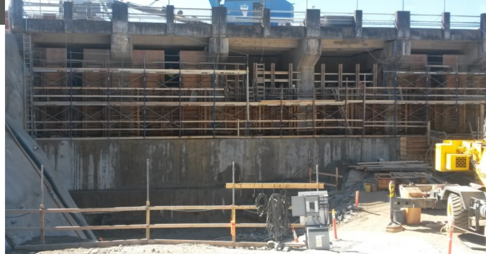
Figure 11: Dam blocks 1, 2 and 3 mass concrete placement is in progress.
