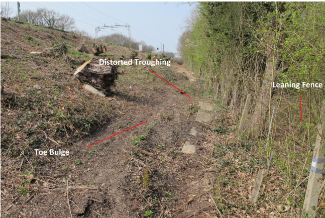
Figure 2B: Evidence of toe bulge which has displaced troughing housing a HV Cable at the embankment toe. The age of the bulge is not known but it is believed to be relatively recent and associated with the current track problems.
