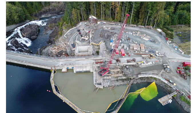
Figure 19: Silt curtain performance after cofferdam removal, INOG structure under construction.
