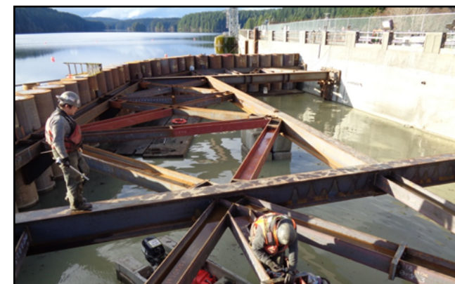
Figure 12: Installation of the cofferdam brace.
