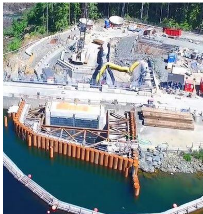
Figure 18: Intake structure before cofferdam removal.
