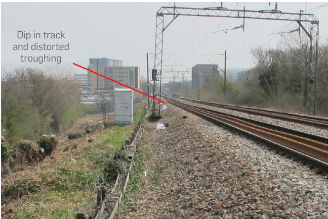
Figure 2A: Cross Section view of the embankment showing the worst area of poor track condition and leaning overhead line. The photograph was taken in summer 2015 and shows the site after removal of large trees with some grow back of grass and small bushes evident.
