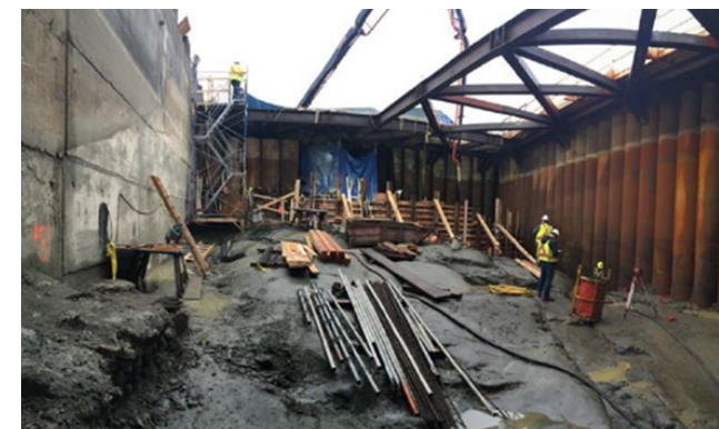
Figure 13: Dewatered cofferdam area.
