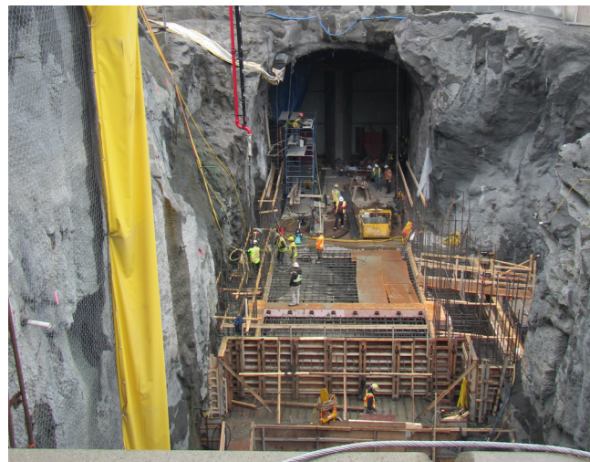
Figure 17b: Excavation of the intake upper bend shaft excavation and construction of intake tunnel
