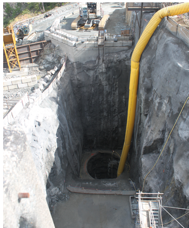
Figure 17a: Excavation of the intake upper bend shaft excavation and construction of intake tunnel
