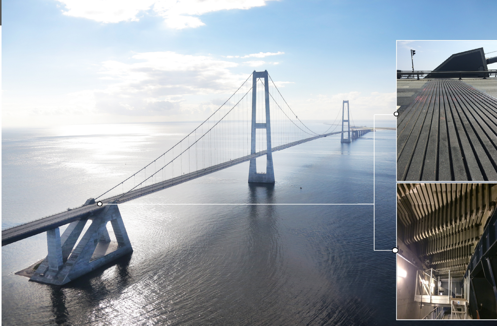
Figure 2: Great Belt East Bridge expansion joint
