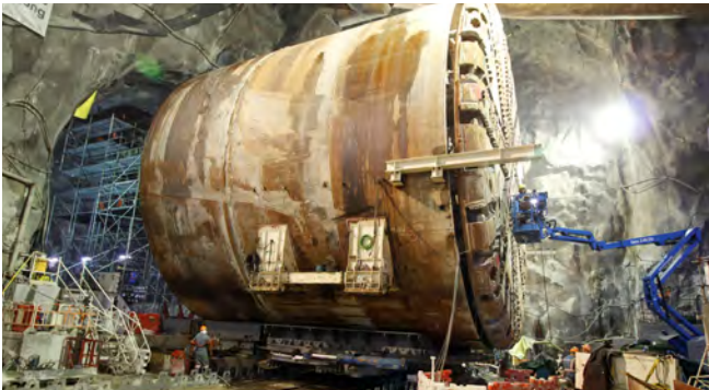
Figure 4a: Photos of TBM U-turning Operation. Photo credits to DHK
