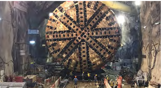
Figure 4b: Photos of TBM U-turning Operation. Photo credits to DHK
