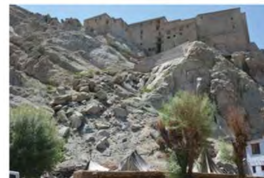
Wedge failure in rock slope below palace
