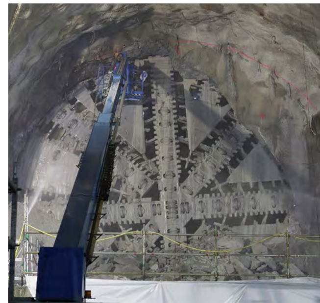
Figure 3b: TBM breakthrough at Southbound Tunnel
