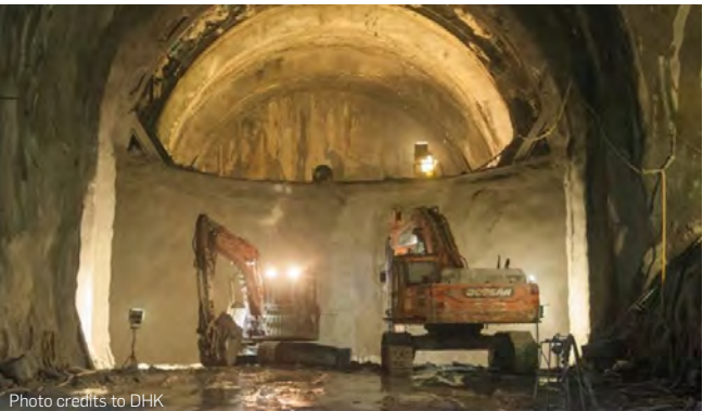
Figure 9: Photos of NB Tunnel – Top heading and bench
