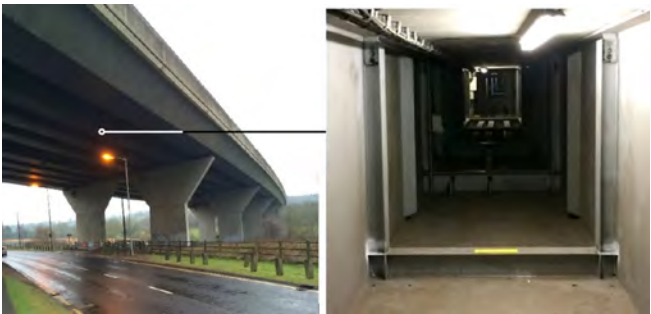
Figure 15: Gade Valley Viaduct and a Typical Internal Crossframe
