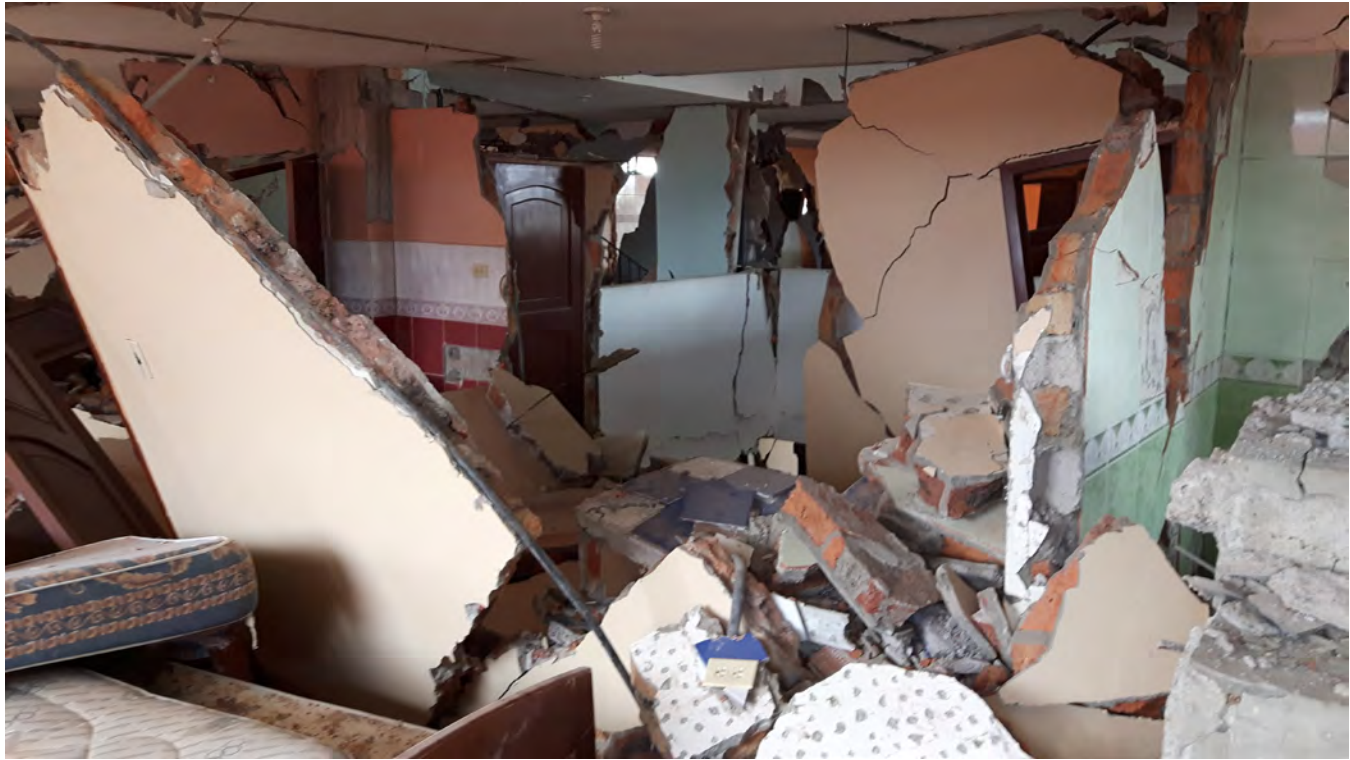
Figure 8. Significant Internal (Non-Structural) Damage Apartments
