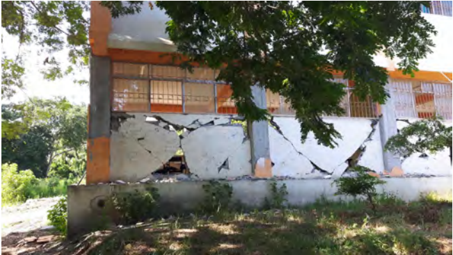
Figure 10. Diagonal Shear Cracks and Damage to External Un-Reinforced Block-Work Walls
