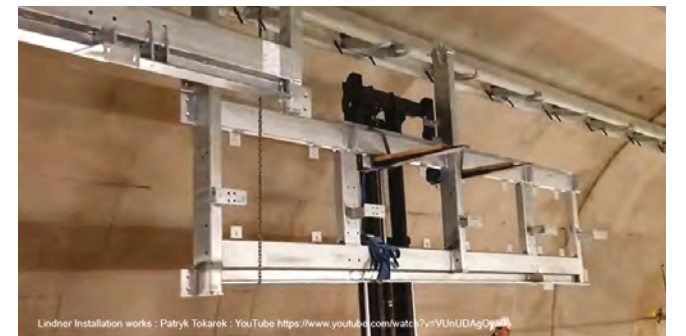
Figure 7: 6m Length of PES Vierendeel Truss Being Lifted Into Place at Farringdon Station (Note Top and Side Alignment Beams Already in Position)
